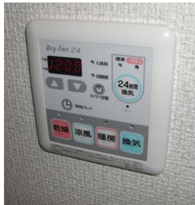
24 hours ventilation system
